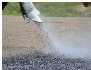
3. Fill: Inject emulsion coated aggregate and fill pothole.
