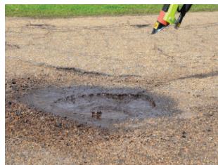
2. Tack: Prep the patch with a coating of emulsion.
