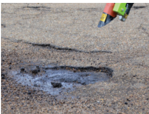
1. Clean: Use high volume low pressure air to clean the patch of debris.
