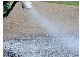
4. Coat: Apply a light coating of clean aggregate and open to traffic.
