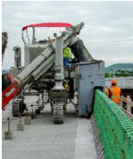
Pouring barrier over rebar cage.
