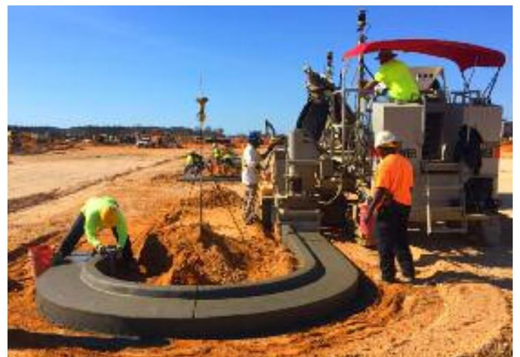
Pouring curb & gutter with 3-D (stringless) control.
