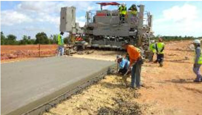
▲ Power Curbers 7700 Multipurpose Slipform Machine Paving
