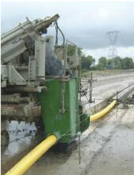
Slotted drain in Uzbekistan showing inflated tube.
